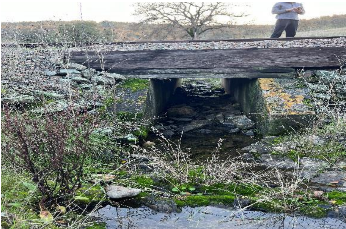
Photo 6: Elevation of bridge, left side of track
