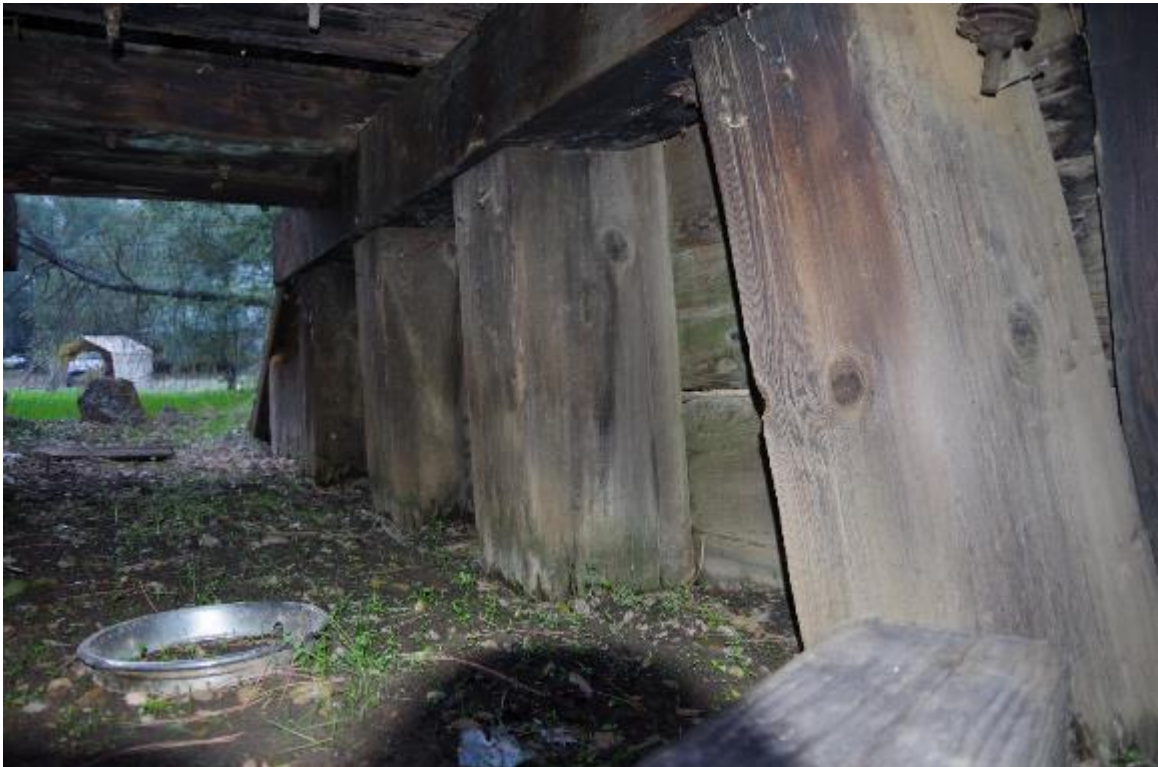
Photo 6: Bent 2 at Abutment 2. All columns are square.
