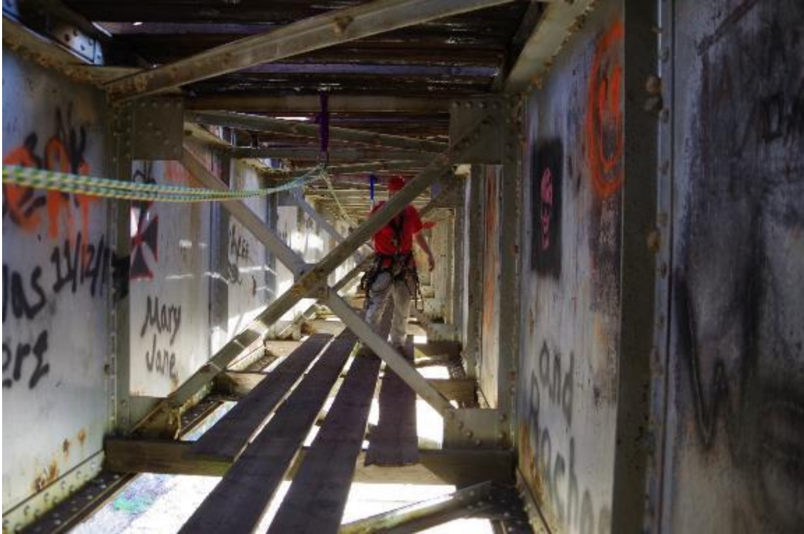
Photo 7: Inside steel girders. Cross lateral bracing shown.
