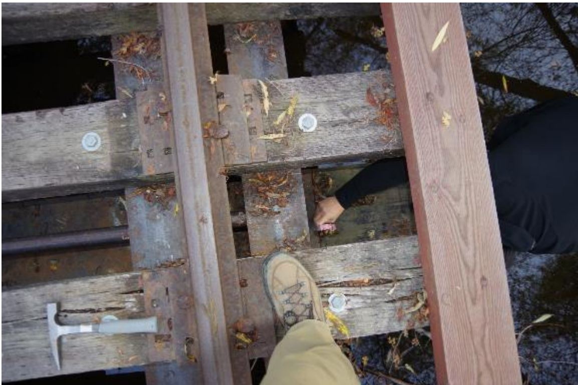
Photo 8: Top view of track above Pier 2
