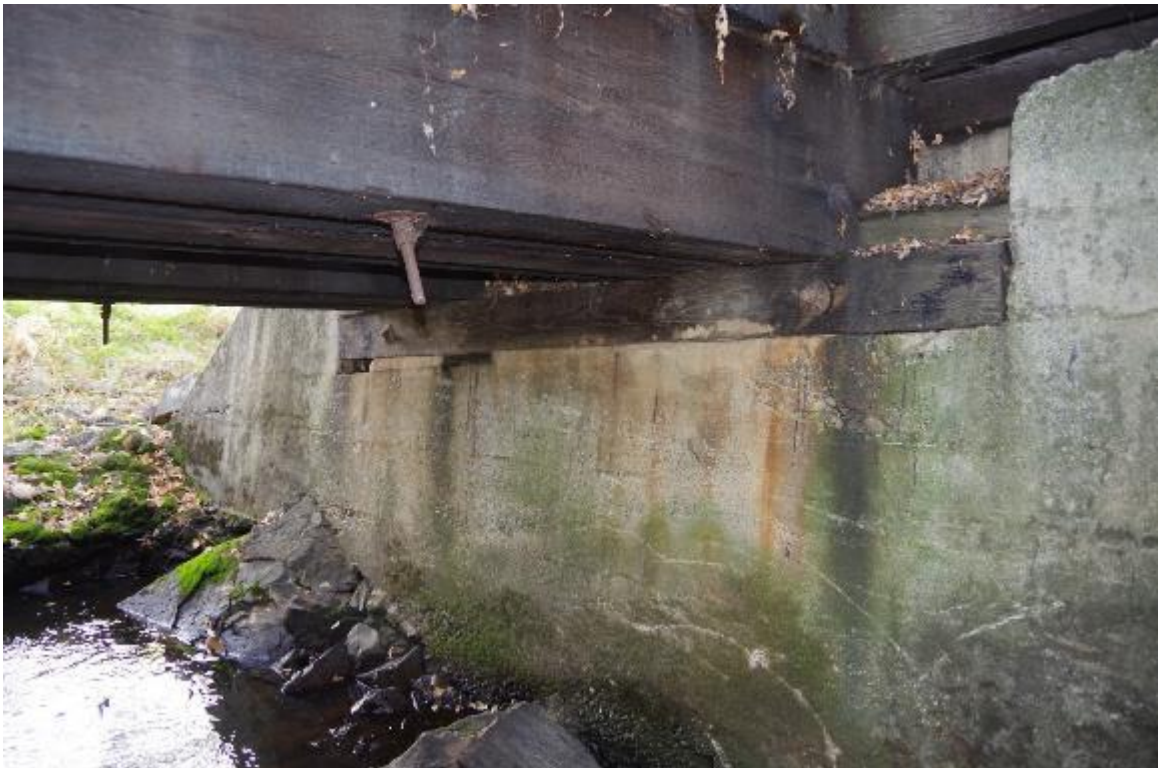
Photo 6: View of Abutment 1 seat.
