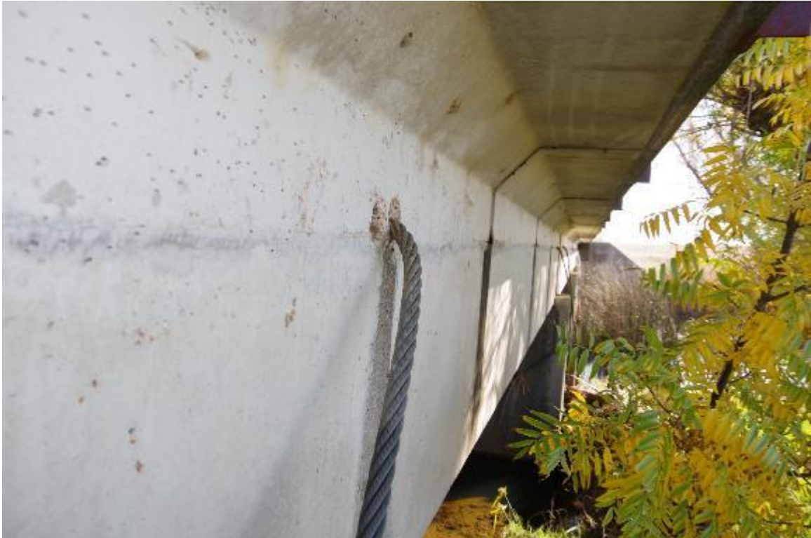
Photo 11: Side view of concrete box culvert.
