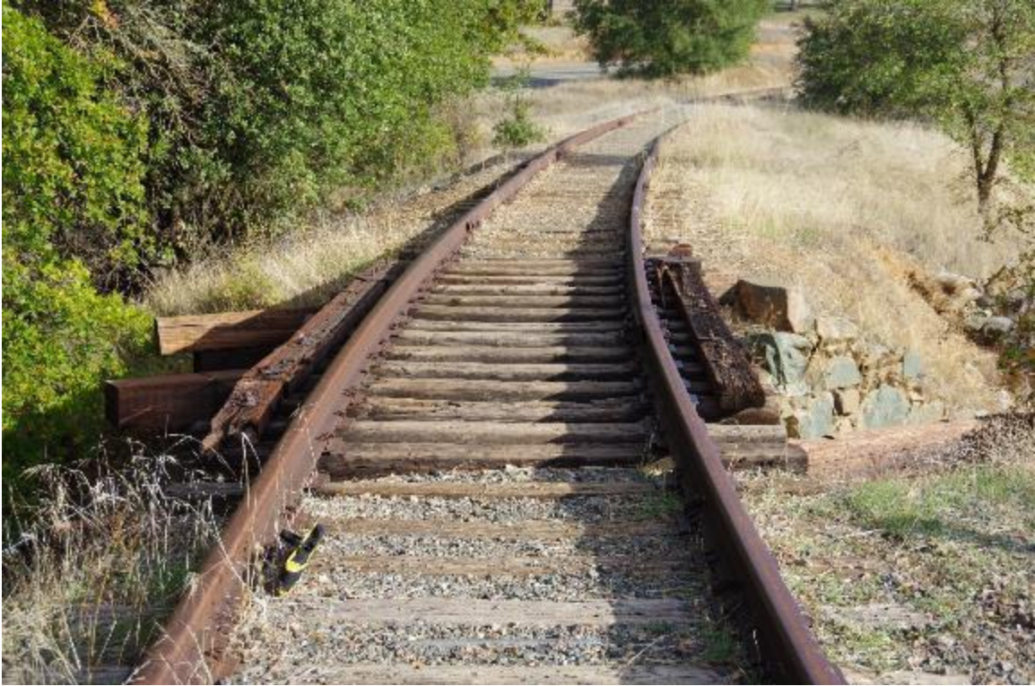
Photo 1: Top view of bridge looking up station
