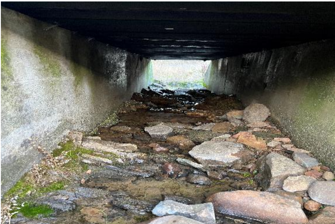
Photo 4: Inside of bridge. Abutment 1 and 2 shown
