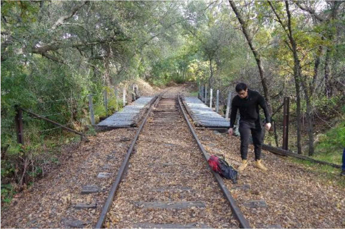
Photo 1: Top view of bridge looking upstation.
