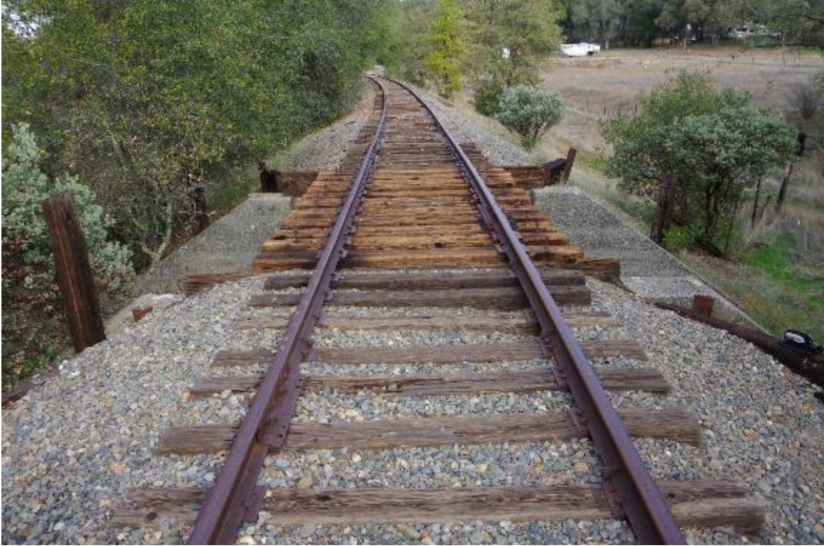
Photo 1: Top view of bridge looking upstation.
