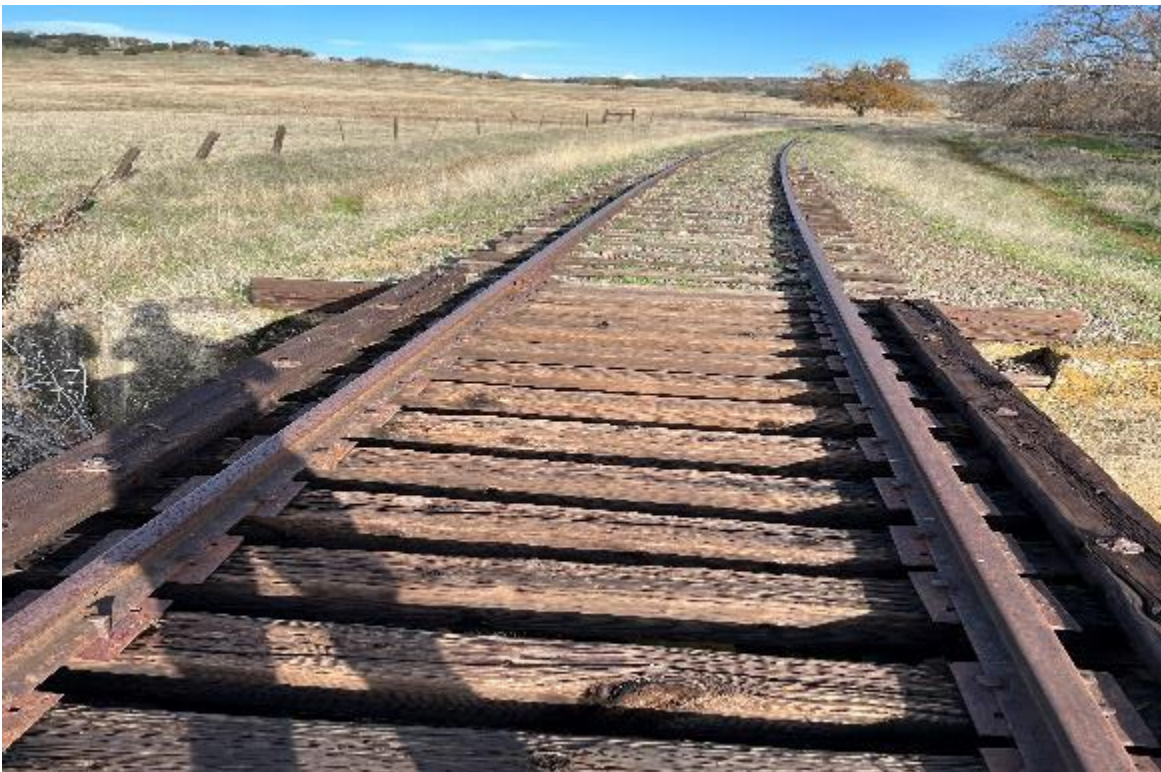
Photo 2: Close up view of top of bridge.
