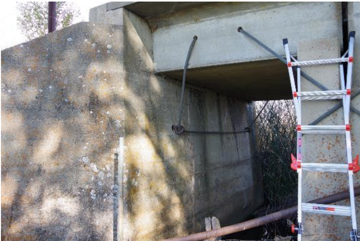
Photo 4: Close up of Span 1 (8'-0"). Shown are Abutment 1 and Pier 2.
