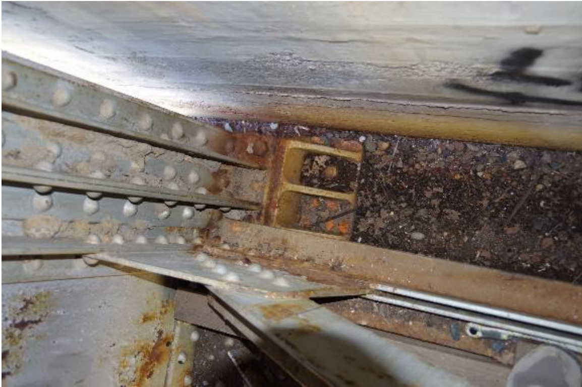
Photo 9: Steel girder connection to concrete seat abutment
