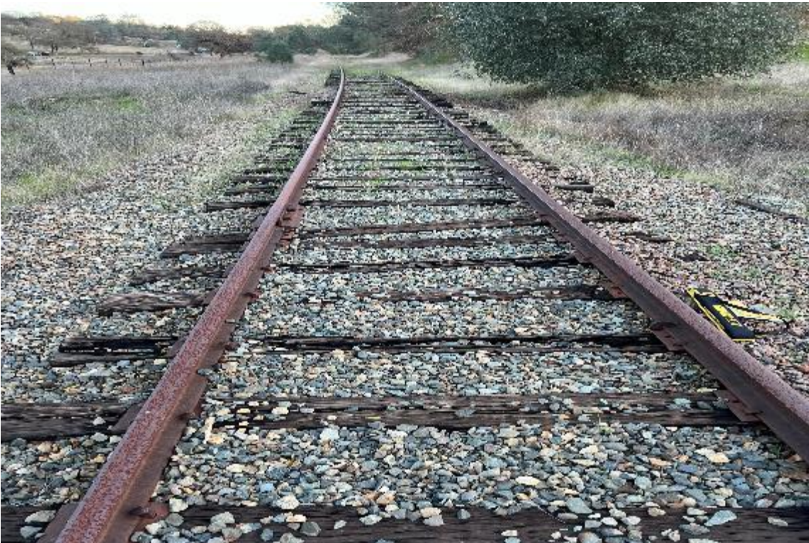
Photo 2: Closeup view of track
