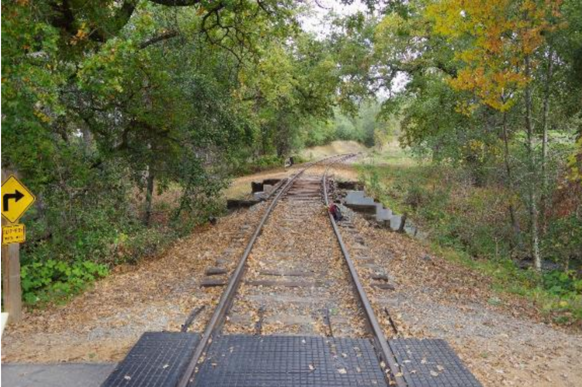
Photo 1: Top view of bridge looking upstation. Pedestrian path located nearby.
