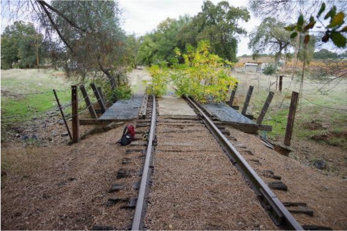
Photo 1: Top view of bridge looking upstation.
