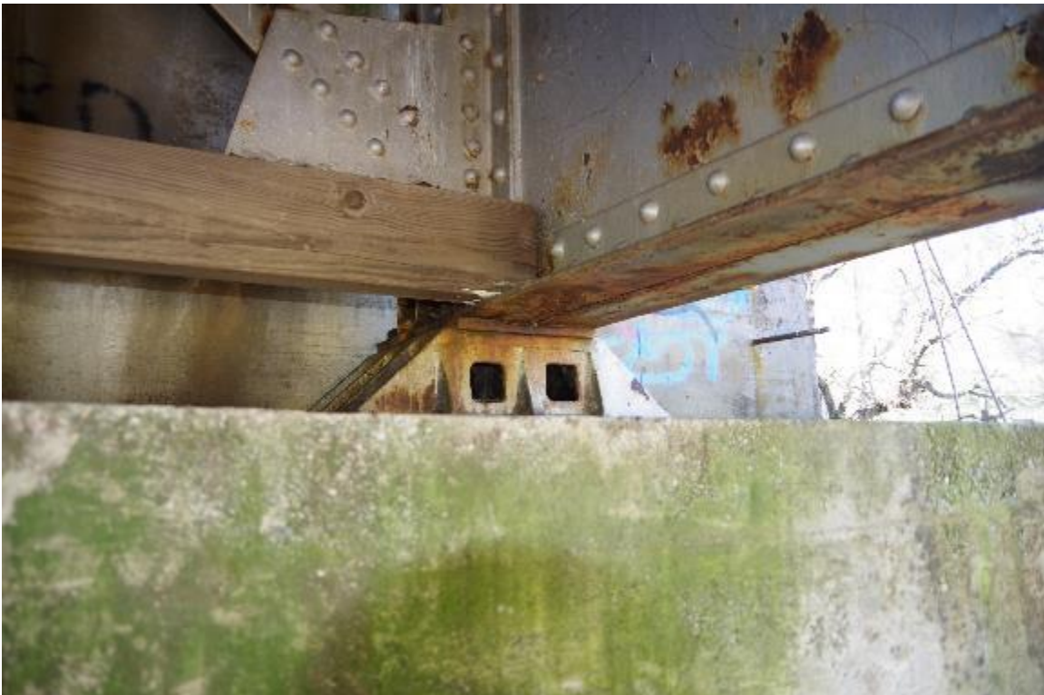
Photo 14: Steel Girder to Concrete Abutment Connection
