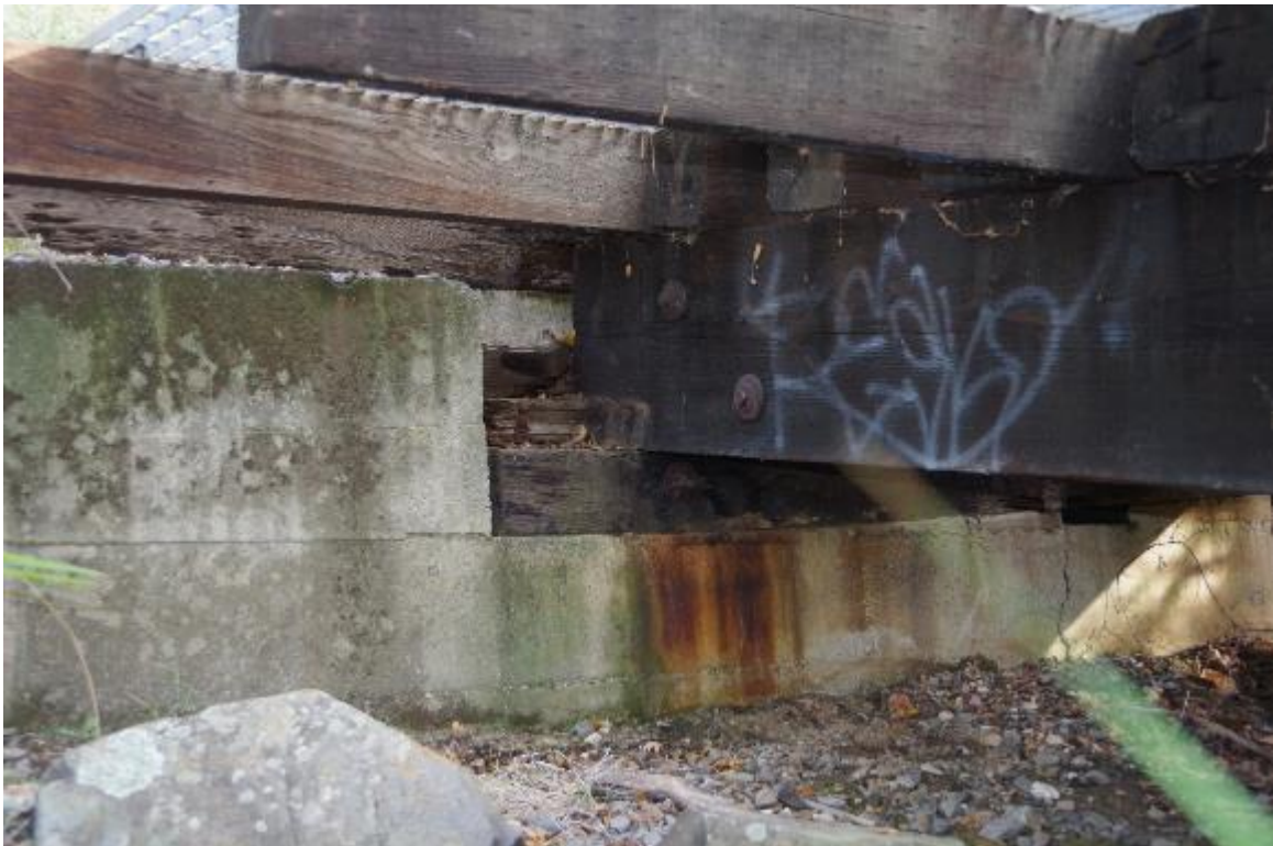
Photo 8: Left side of Abutment 2.
