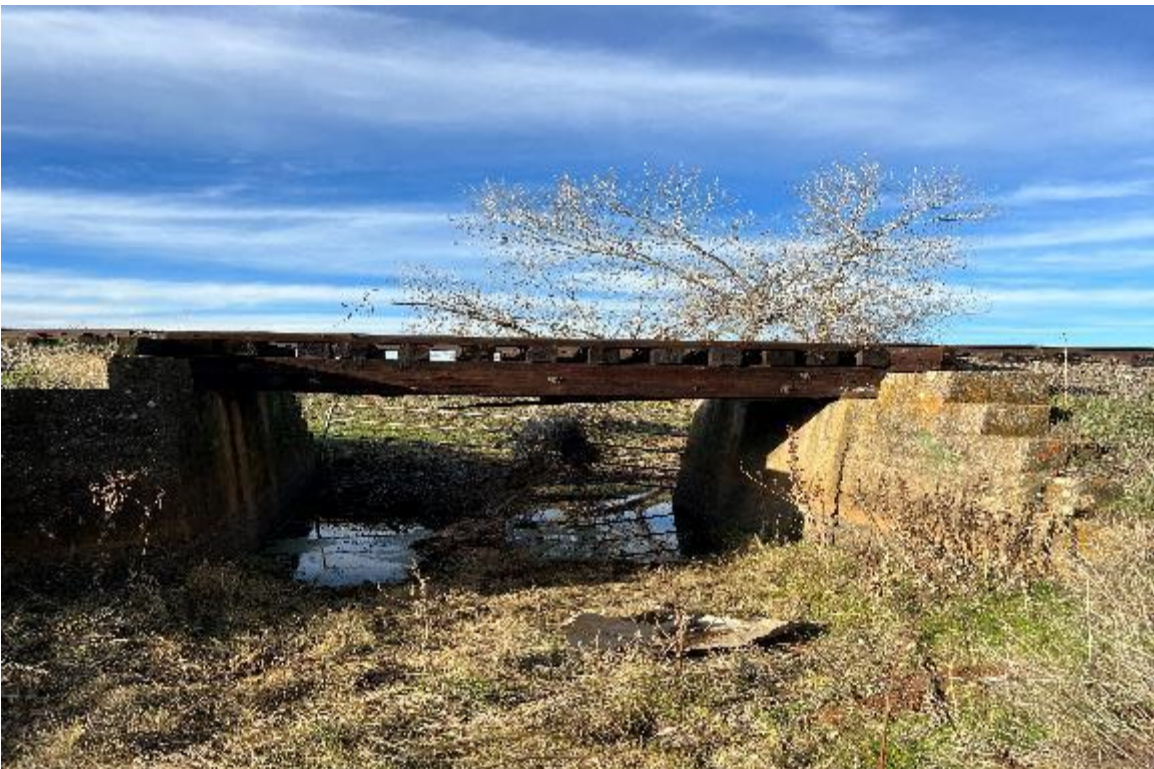
Photo 4: Elevation view of bridge from the right side of the track.
