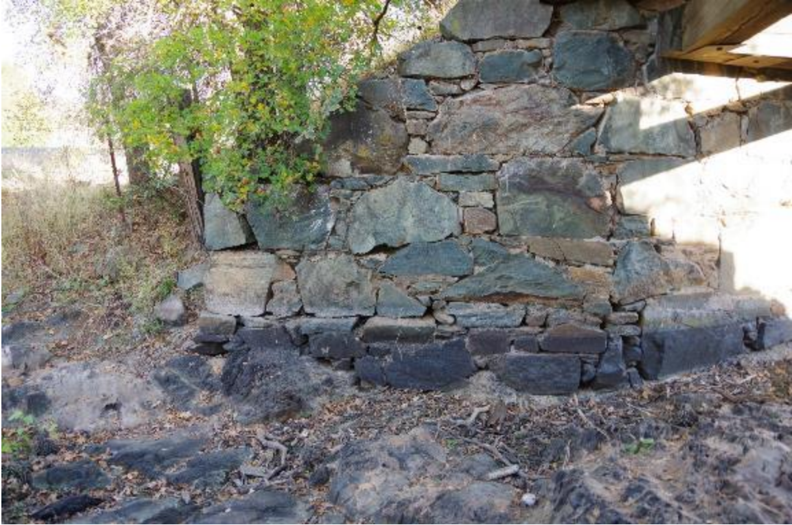
Photo 7: Left side view of abutment 2. Stone abutment, in fair condition.
