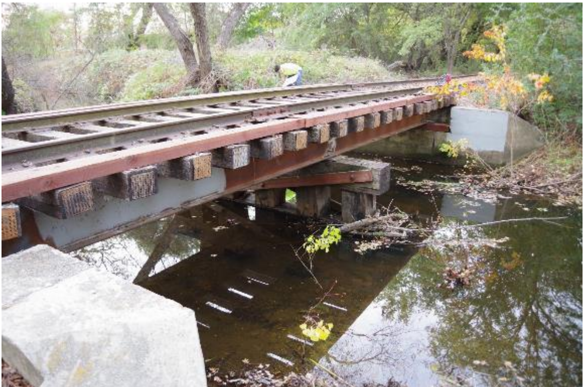
Photo 2: Bridge elevation view, west side of bridge over Willow Creek.
