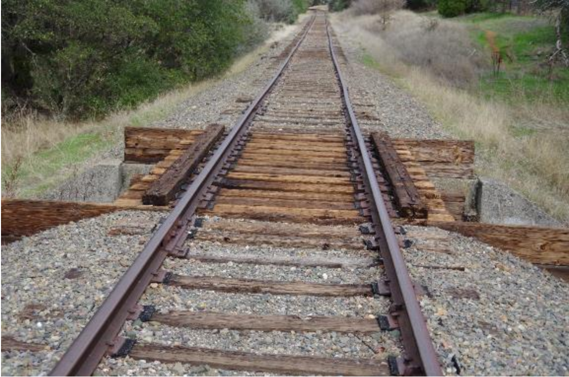
Photo 1: Top view of bridge looking upstation.
