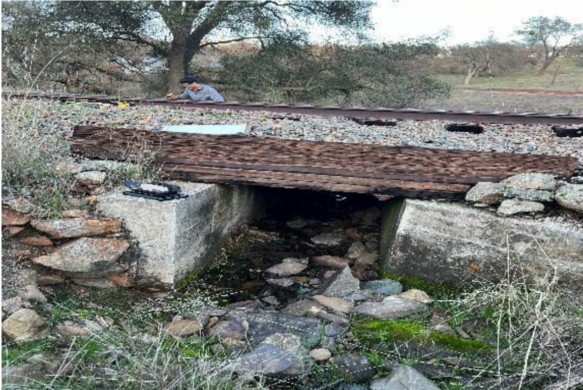
Photo 3: Elevation view of bridge, right side of track
