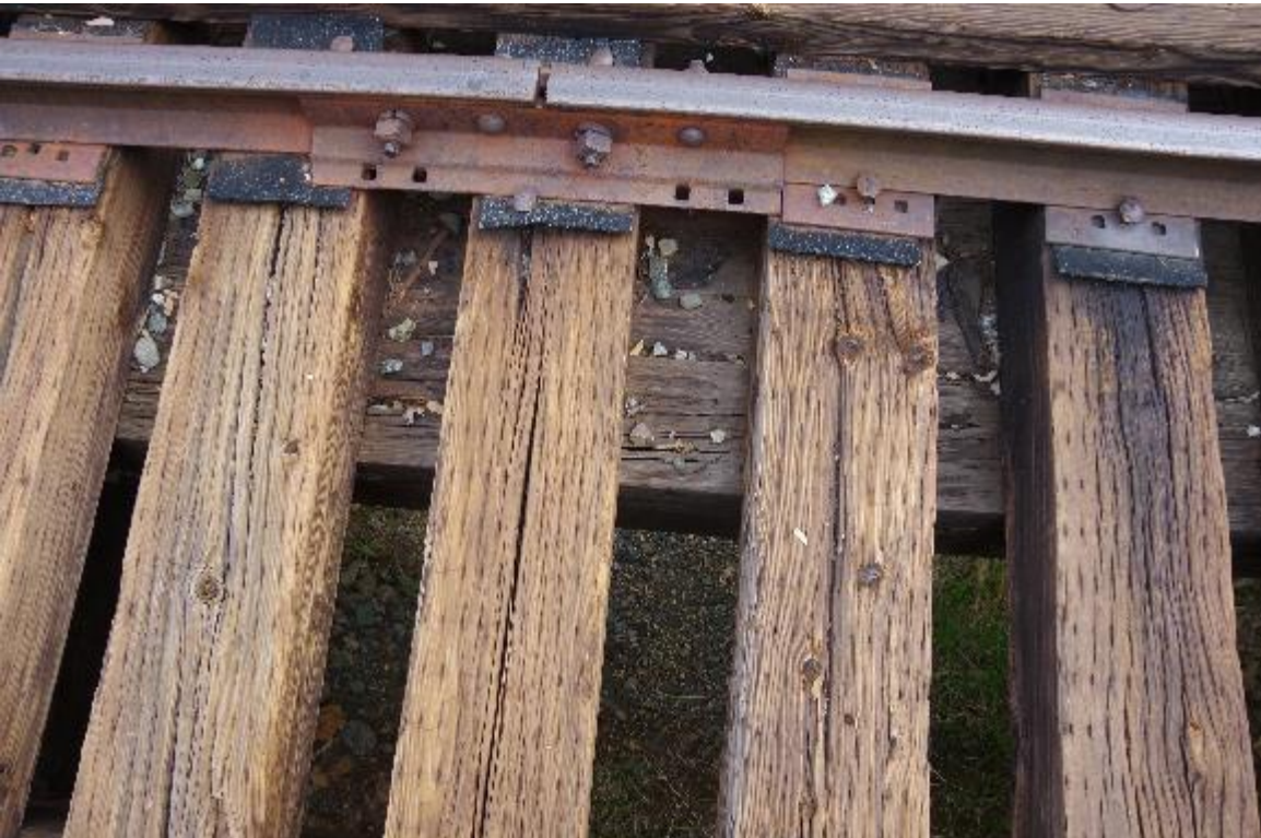
Photo 6: Closeup view of railroad ties and steel track.
