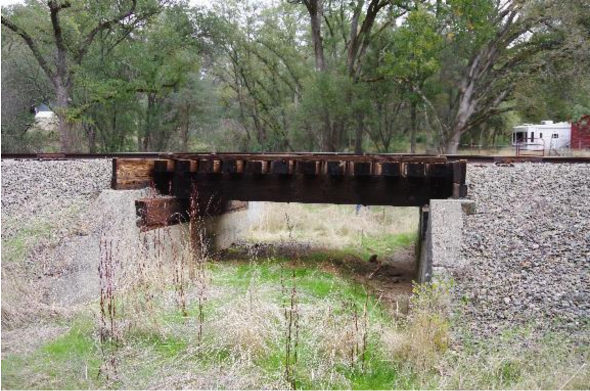
Photo 5: Elevation view of bridge on the left side of the track.
