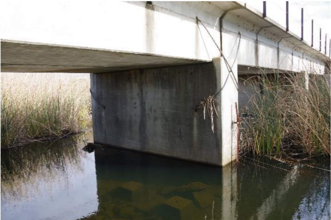
Photo 6: View of Pier 3.
