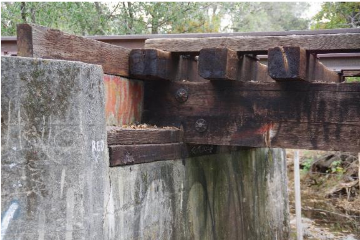
Photo 9: Timber girder to abutment 5 connection.
