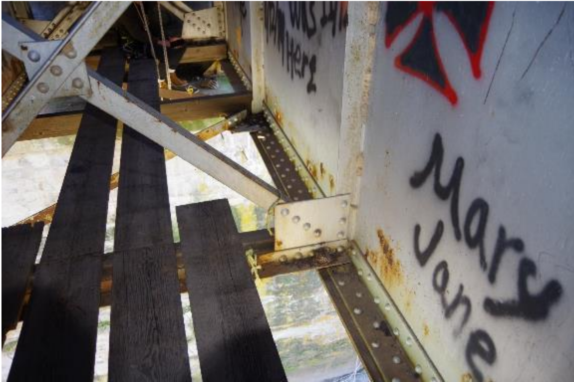
Photo 11: Vertical Gusset Plate Connection
