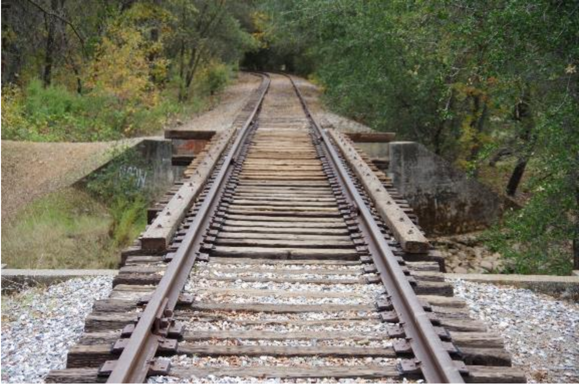
Photo 1: Top view of bridge looking upstation.
