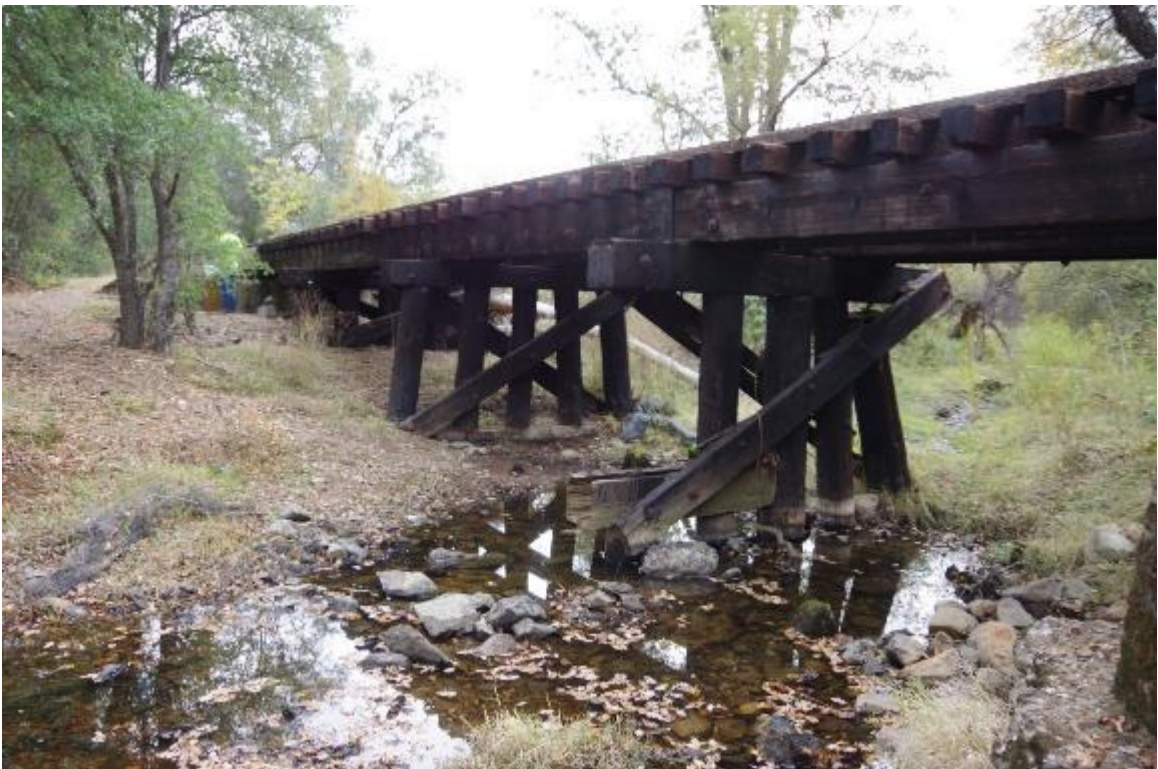
Photo 2: Bridge elevation at left side of track. Pier 2 and 3 shown.
