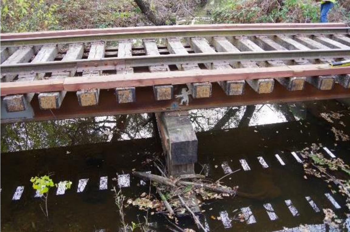
Photo 3: Pier 2 view from west side of bridge
