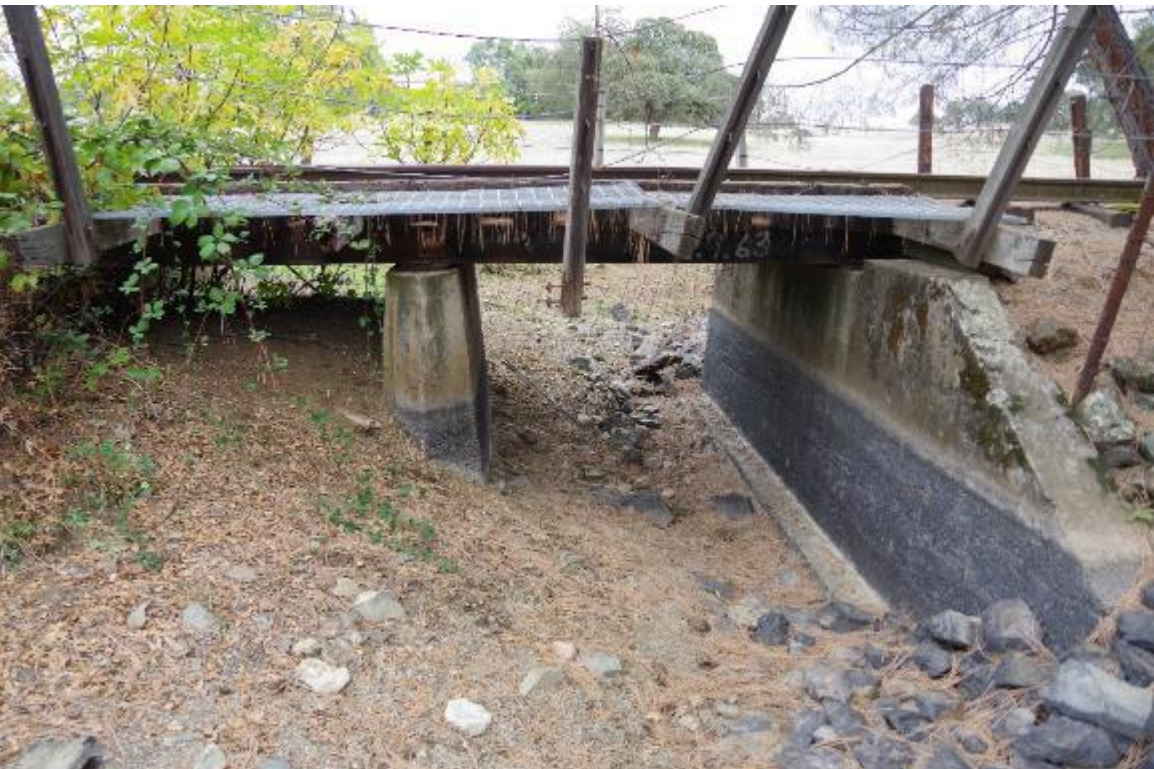
Photo 2: Bridge elevation view, left side of track.
