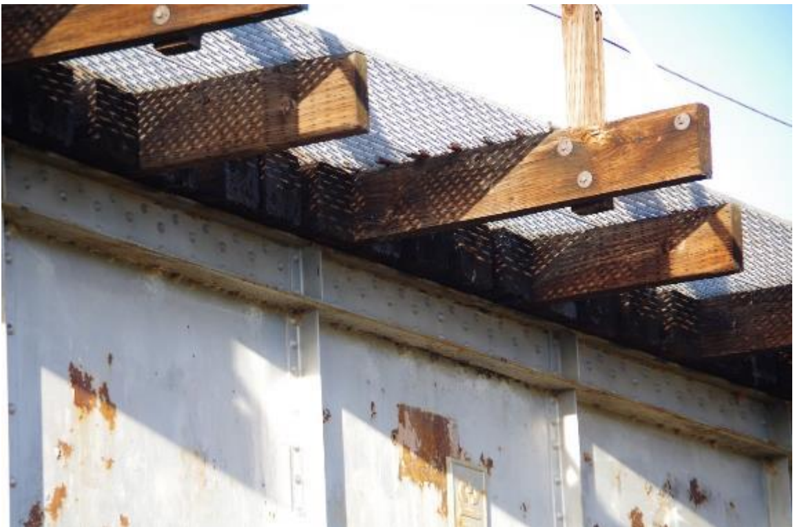
Photo 4: Closeup view of steel girder, railroad ties, and walkway supports.
