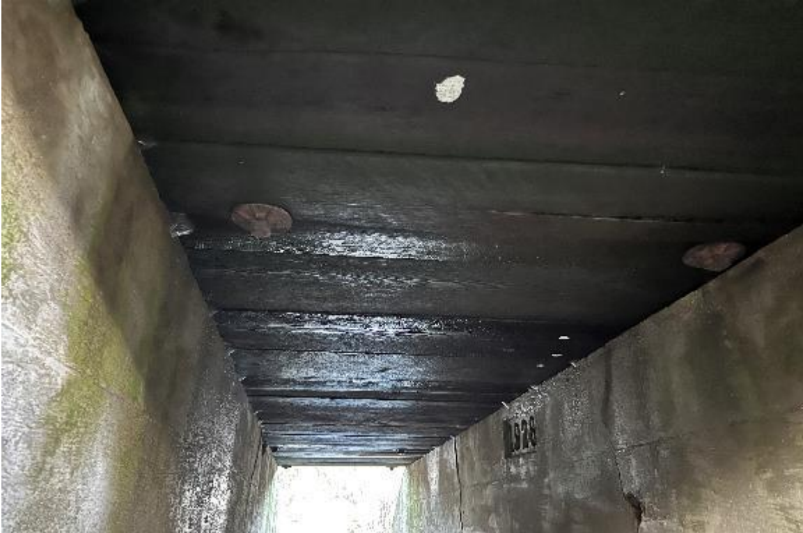
Photo 5: Timber beams along width of the bridge
