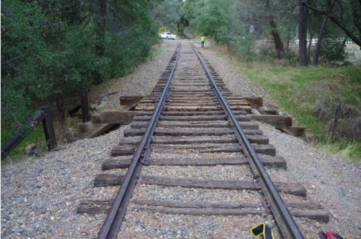
Photo 1: Top view of bridge looking upstation.
