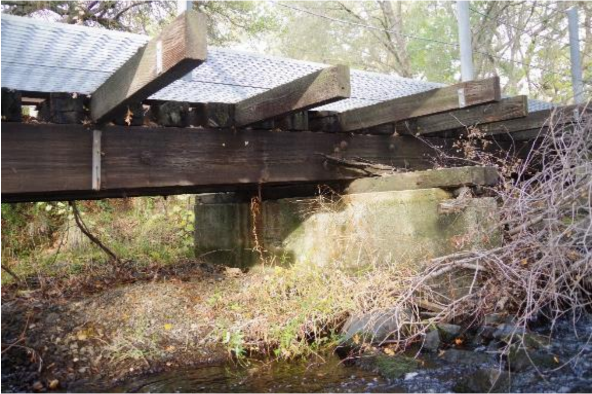
Photo 11: View of Pier 3.
