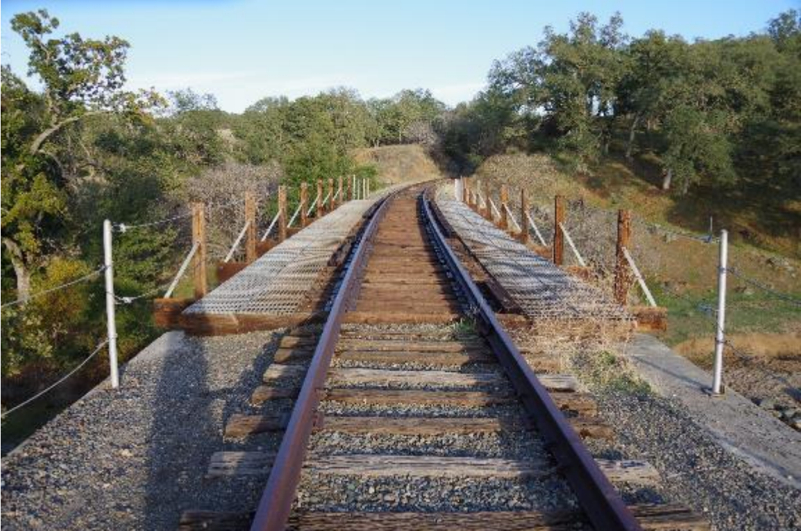
Photo 1: Top view of bridge looking upstation
