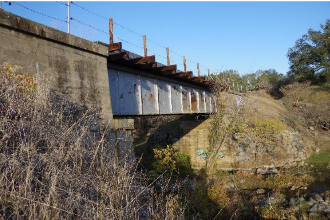
Photo 2: Bridge elevation view, right side of bridge. Abutment 1 & 2 shown.
