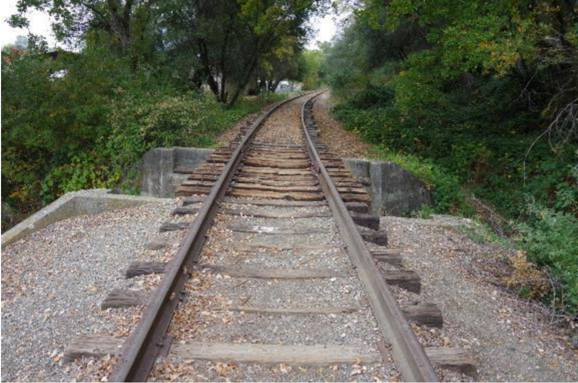
Photo 1: Top view of bridge looking upstation.
