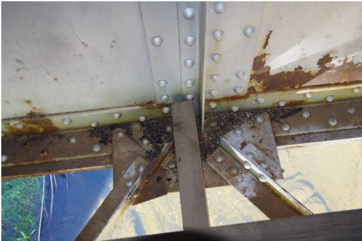
Photo 10: Gusset Plate Connection
