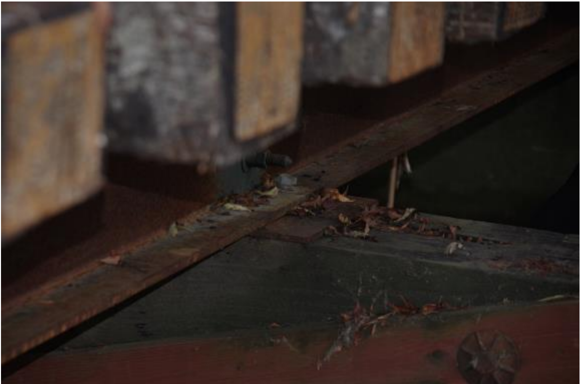
Photo 6: Typical steel girder to timber bent connection (Pier 2)
