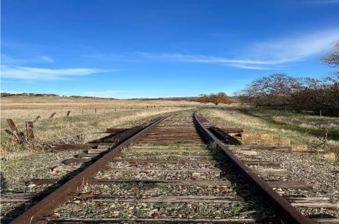
Photo 1: Top view of bridge with track, looking upstation
