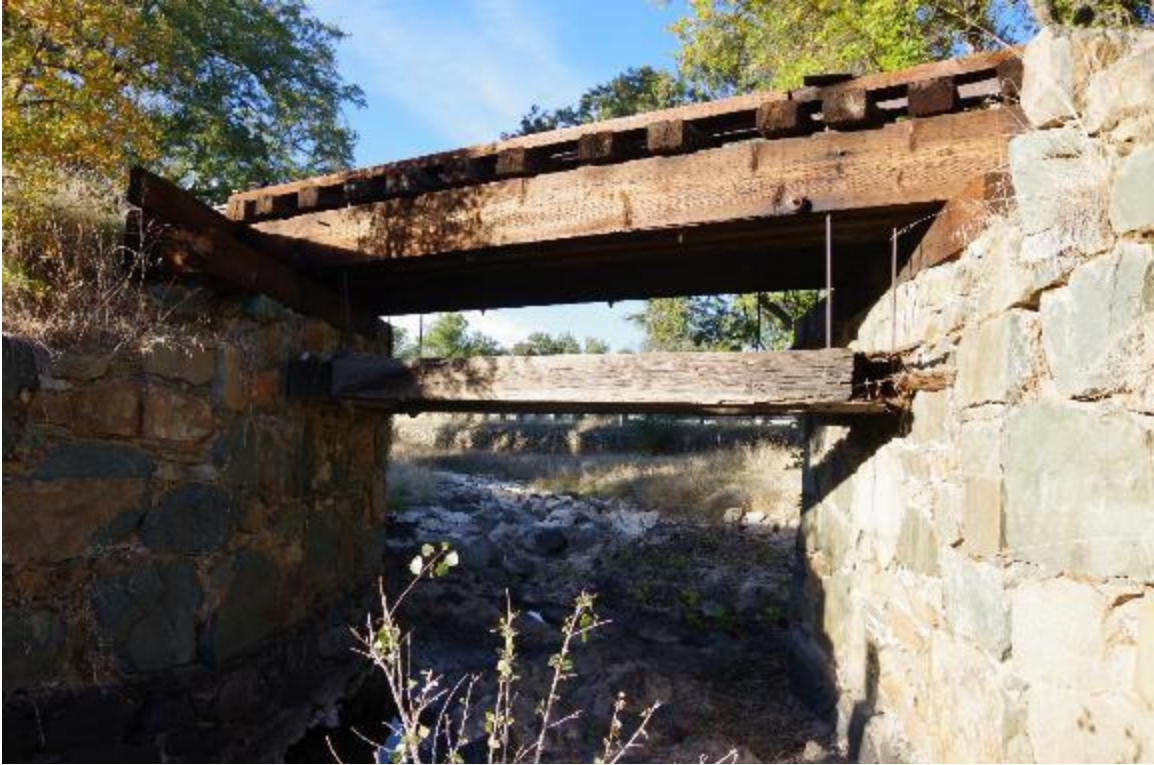
Photo 3: Bridge elevation view from right side of track.
