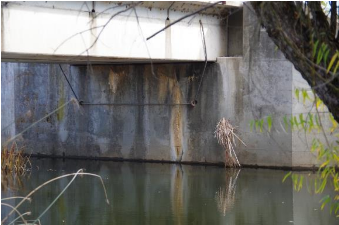
Photo 8: View of Abutment 5. Seismic restrainer shown.
