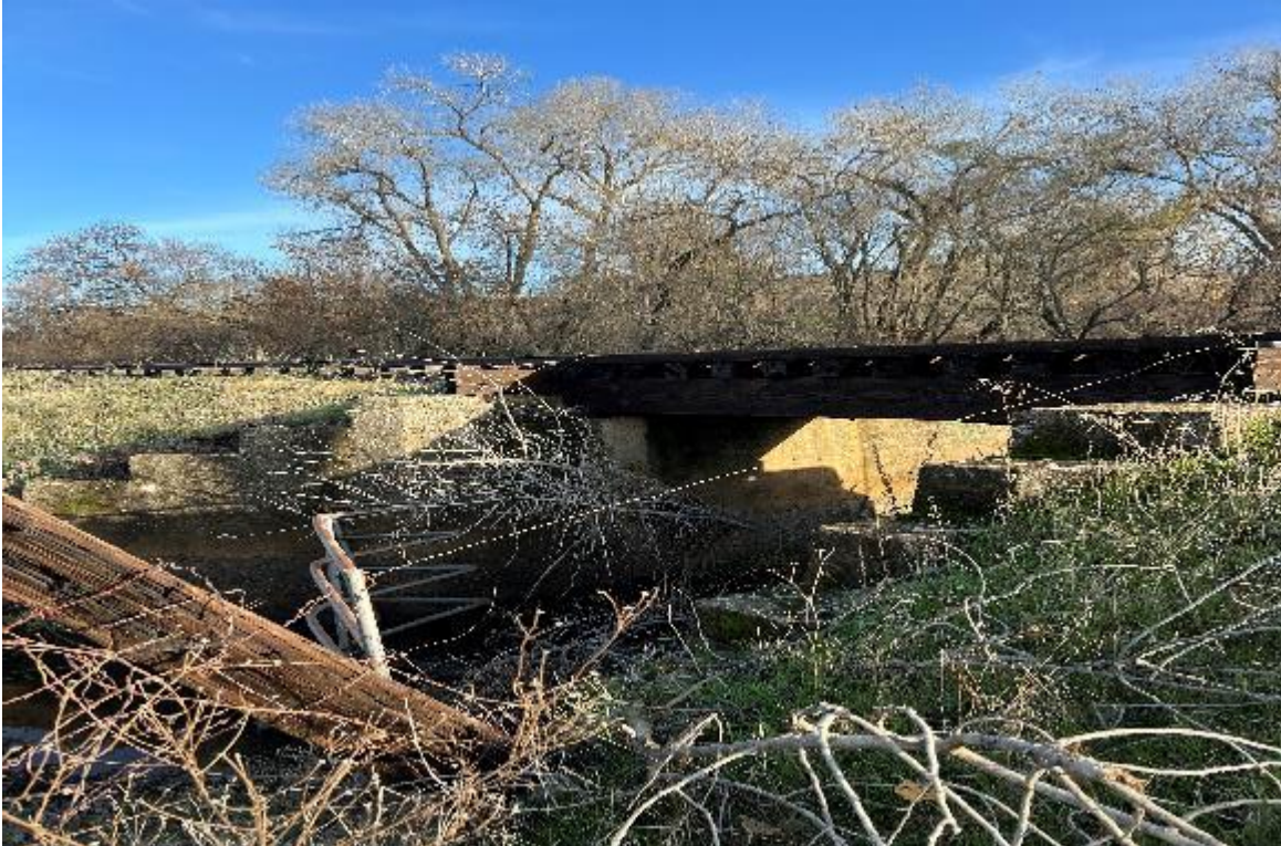
Photo 7: Bridge elevation view from left side of track.
