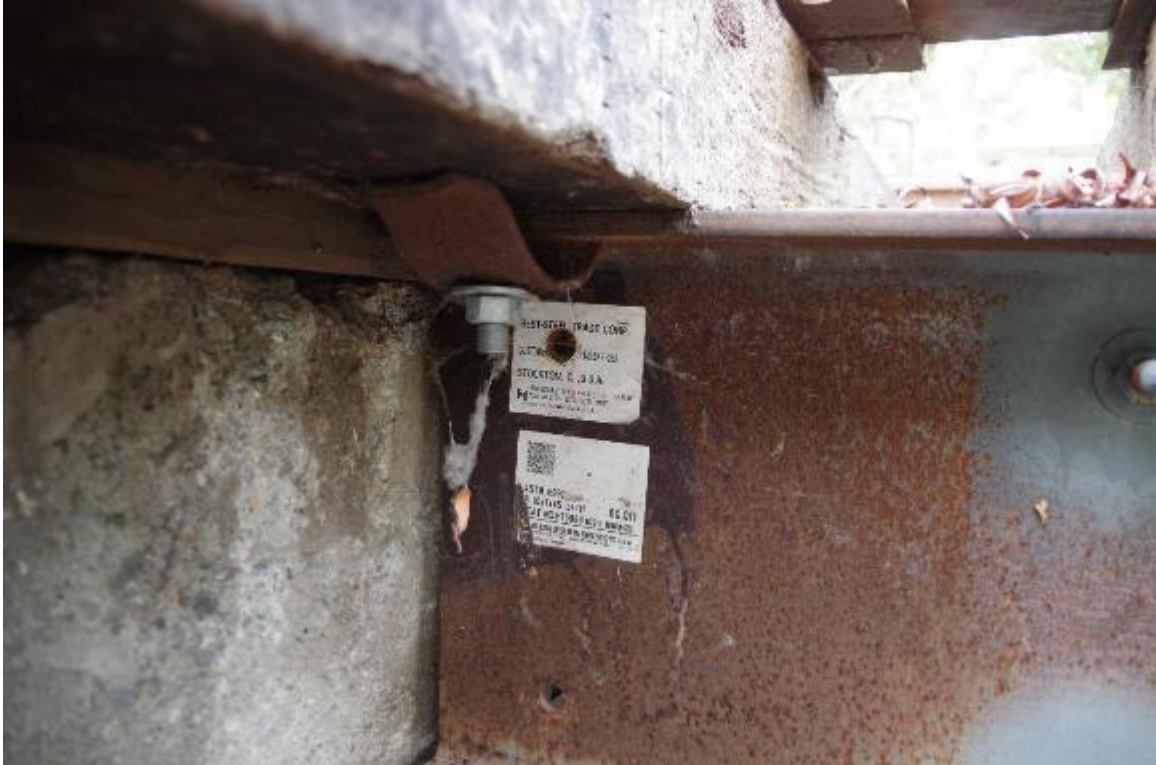
Photo 7: Steel girder to Abutment connection
