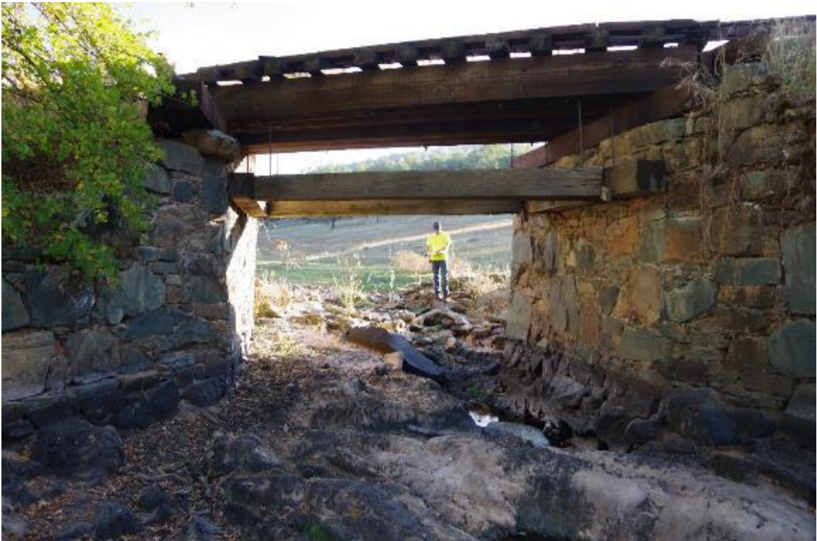
Photo 2: Bridge elevation view from left side of track.
