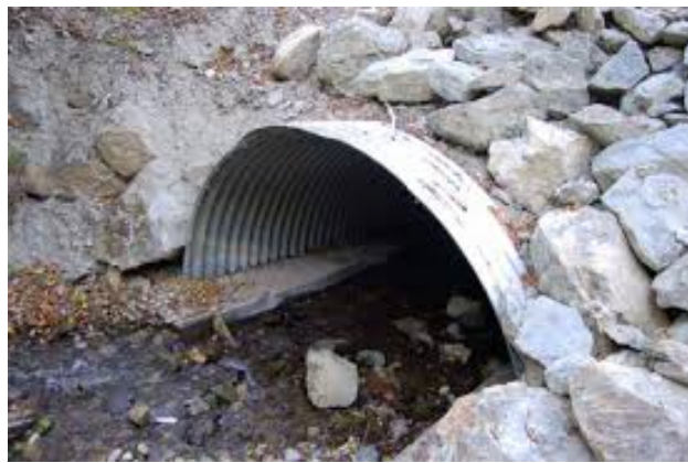
Figure 4 — Multi-plate Structure, photograph from www.fhwa.dot.gov
