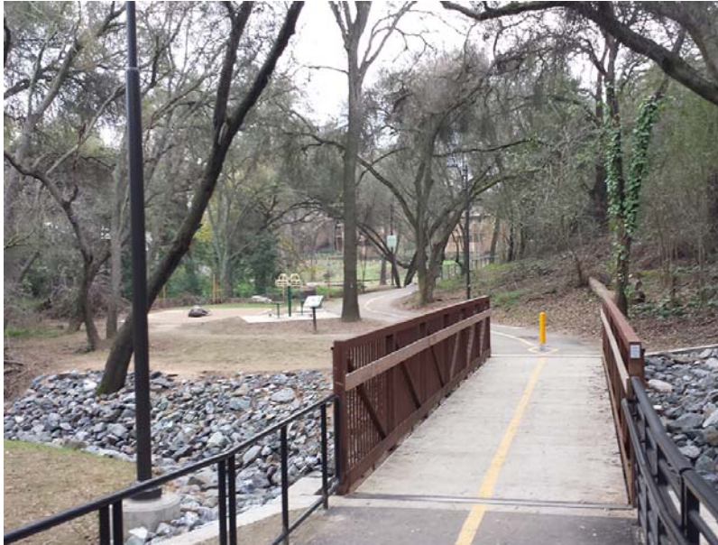
Figure 5 — Prefabricated Steel Bridge with Concrete Deck photograph by Foothill Associates
