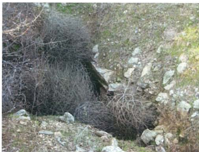
Feature 56: This feature is a greenstone culvert. Facing N. Frame 3430.
