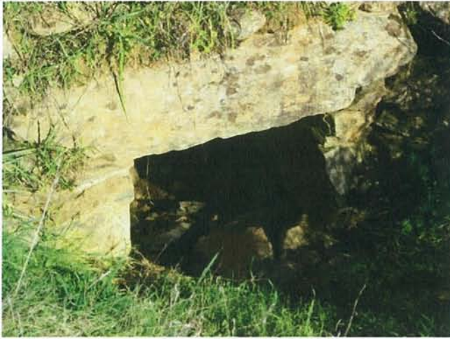
Feature 41: This feature is a square greenstone culvert. Facing E. Frame 3410.
