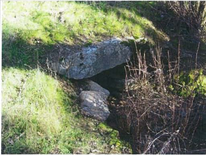
Feature 45: This feature is a stacked greenstone culvert. Facing ESE. Frame 3314.
