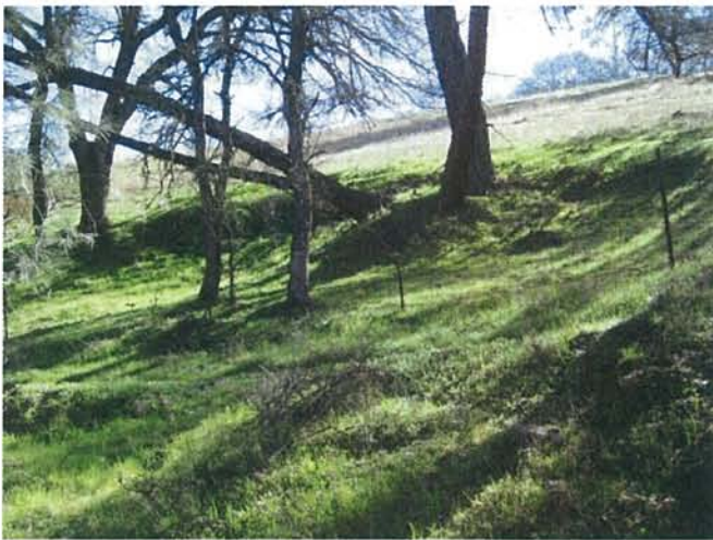
Feature 35: This feature is a large kidney shaped borrow pit for the railroad. It is 36 feet wide south east to north west, and 63 feet long south west to north east. Facing E. Frame 3390.
