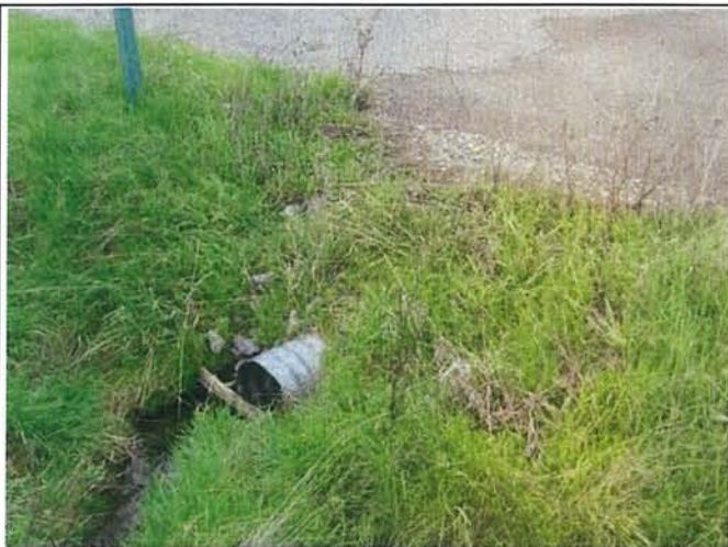
Feature 1: This feature is a steel culvert. Facing S. Frame 3333.
