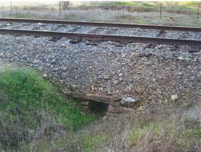
Feature 59: This feature is a very small greenstone culvert. Facing NE. Frame 3434.
