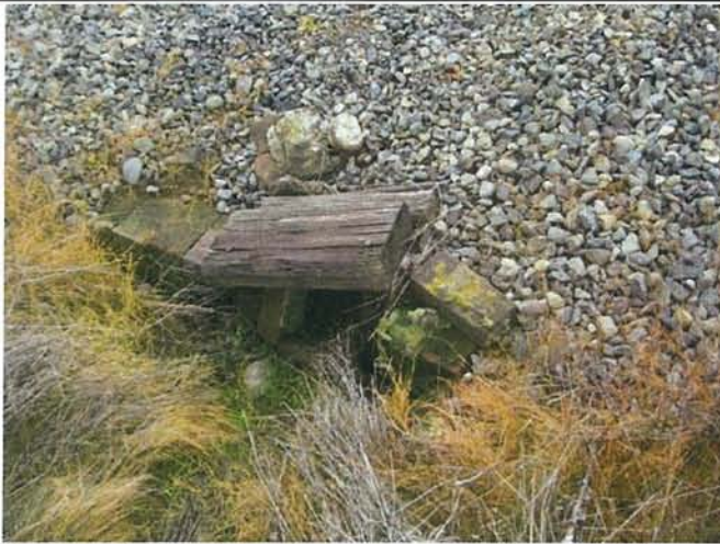
Feature 25: This feature is a wooden culvert surrounded by brick. Facing S. Frame 3336.
