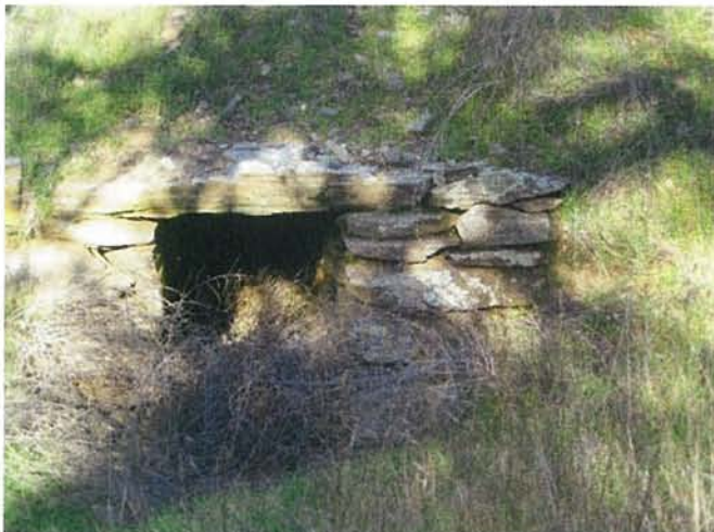
Feature 51: Large rectangular stacked greenstone culvert. Facing N. Frame 3420.
