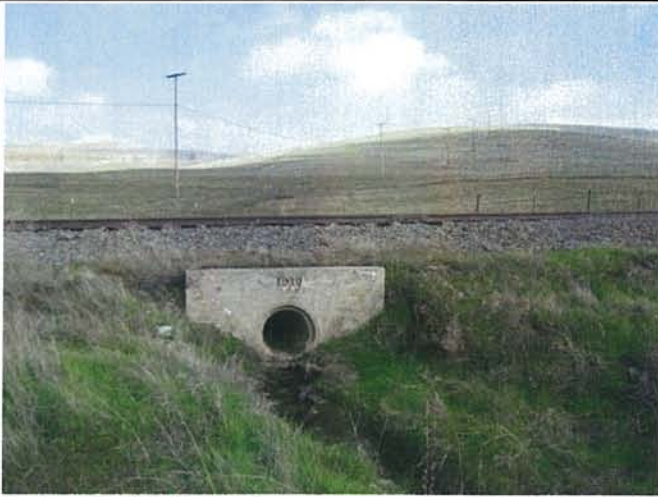
Feature 5: This feature is a concrete culvert "1910". Facing E. Frame 3303.
