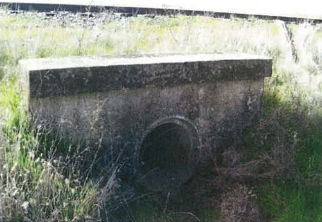
Feature 71: This feature is a poured concrete culvert. Facing SW. Frame 3470.
