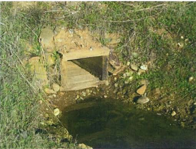
Feature 31: This feature is a square wooden culvert with fragments of clay pipe adjacent to it. Facing E. Frame 3356.
