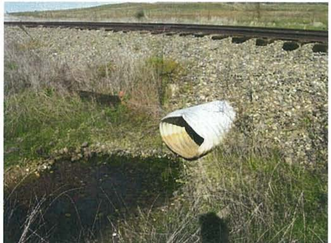
Feature 76: This feature is a corrugated metal culvert. Facing N. Frame 3476.
