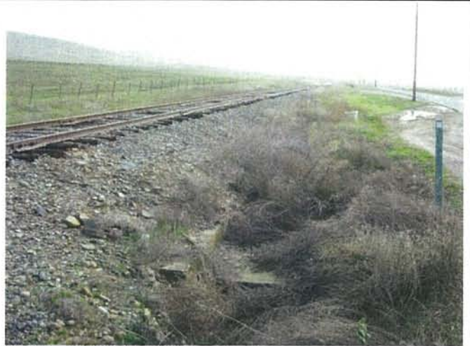
Feature 2: This feature is a concrete capped culvert. Facing SE. Frame 3299.
