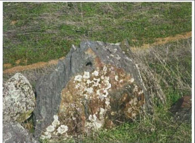
Feature 66: This feature is an anchor point drilled into a local boulder. Facing NNW. Frame 3453.
