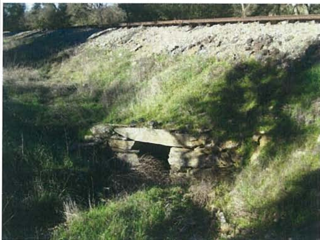
Feature 55: This feature is a stacked greenstone culvert. Facing N. Frame 3327.
