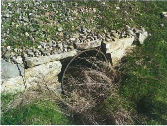
Feature 85: This feature is stacked greenstone surrounded an iron pipe culvert. Facing E. Frame 3493.
