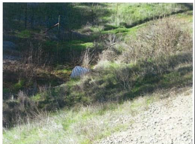
Feature 40: This feature is a corrugated metal culvert. Facing W. Frame 3409.
