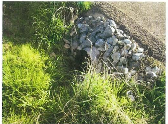
Feature 8: This feature is a galvanized metal culvert. Facing S. Frame 3355.
