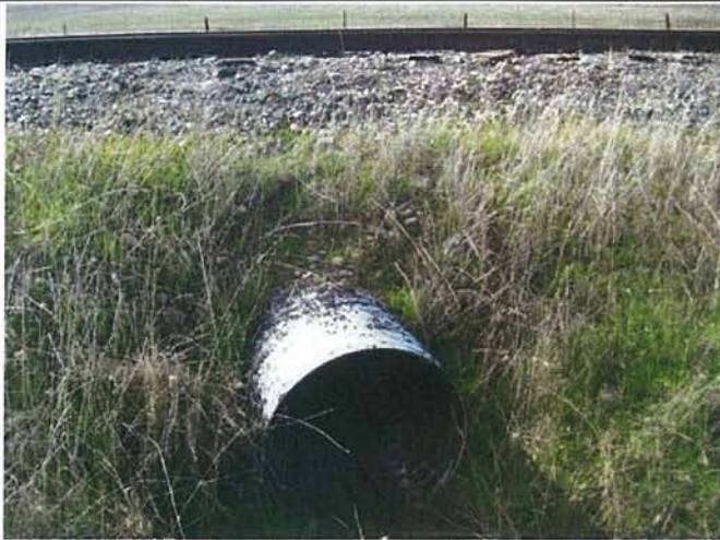
Feature 73: This feature is a corrugated metal culvert. Facing SW. Frame 3472.
