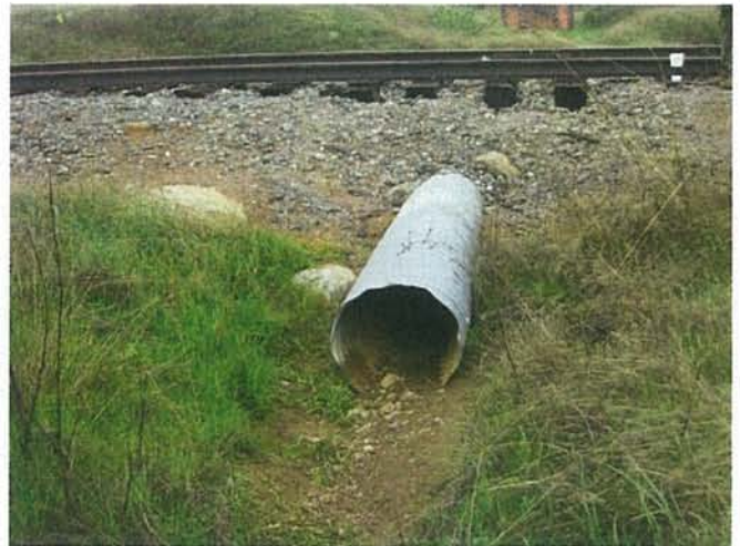
Feature 10: This feature is a USS copper steel corrugated culvert with "6/2/83" stamped on it.
