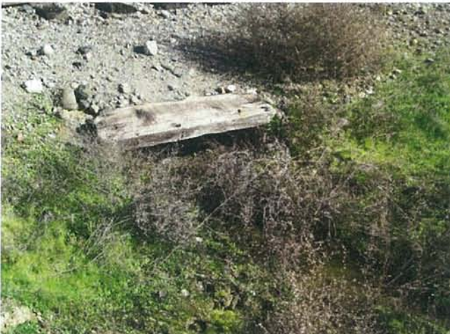
Feature 83: This feature is a shallow wooden culvert. Facing E. Frame 3487.
