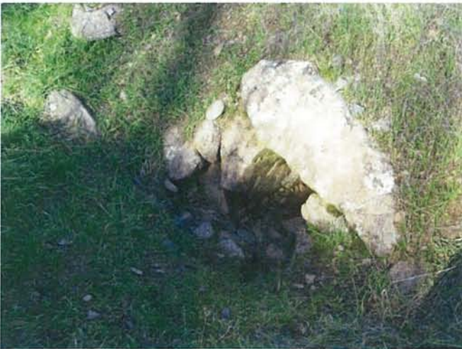
Feature 43: This feature is a square greenstone culvert. Facing N. Frame 3412.
