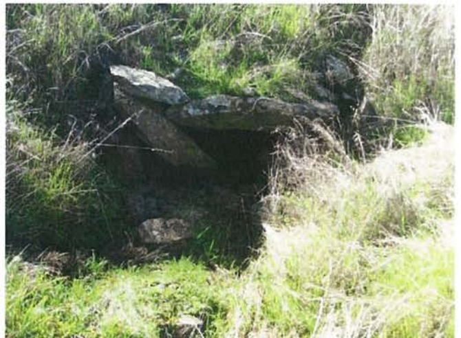
Feature 68: This feature is a stone culvert. Facing S. Frame 3457.
