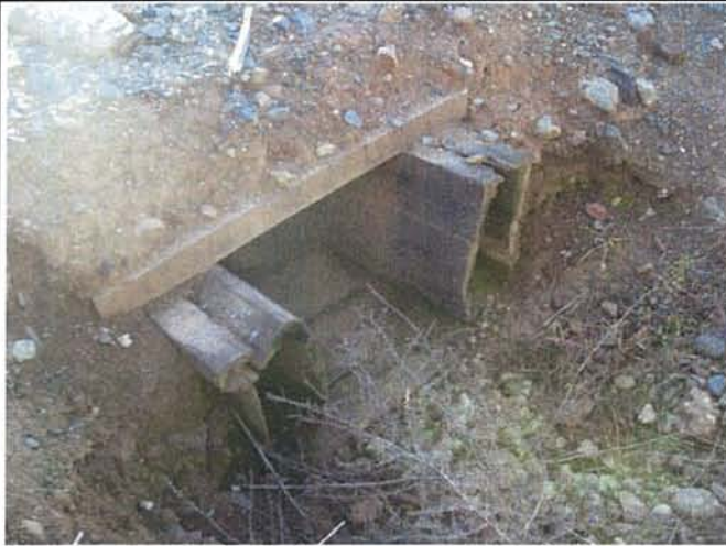
Feature 33: This feature is a square wooden culvert. Facing W. Frame 3360.
