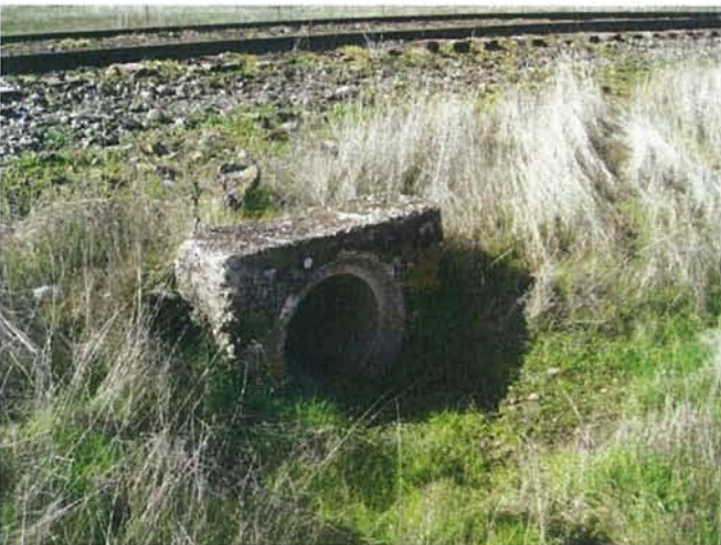
Feature 79: This feature is poured concrete culvert. Facing NW. Frame 3479.
