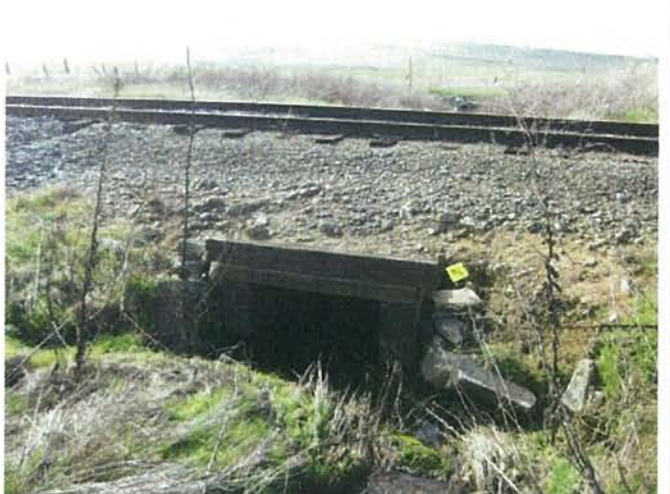
Feature 4: This feature is a timber culvert. Facing W. Frame 3302.
