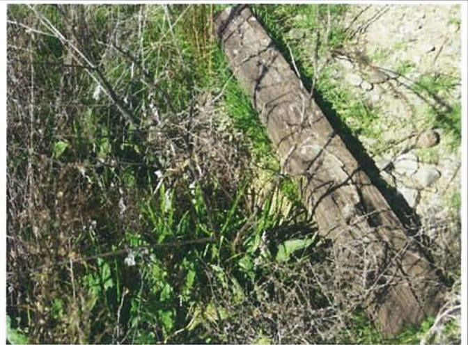
Feature 82: This feature is a shallow greenstone culvert. Facing N. Frame 3485.
