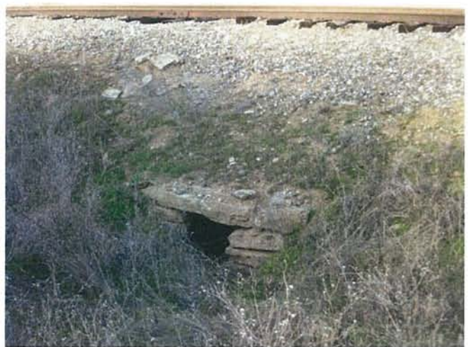
Feature 60: This feature is a stacked greenstone culvert. Facing N. Frame 3435.
