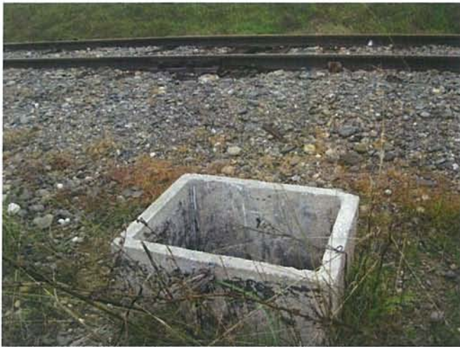
Feature 13: This feature is a concrete default detector box with attached wiring in background, and plastic sheathed wiring attached to the railroad track. There are wire nails and wood at the bottom of the box. Facing N. Frame 3317.
