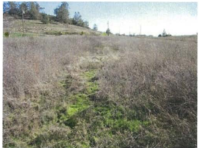
Siding bed on the N side of the track. Facing SE. Frame 3404.
