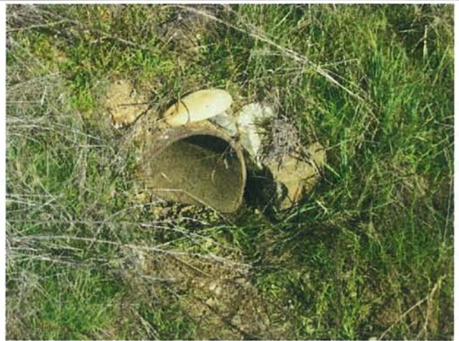
Feature 30: This feature is a concrete cylindrical culvert. Facing E. Frame 3353.
