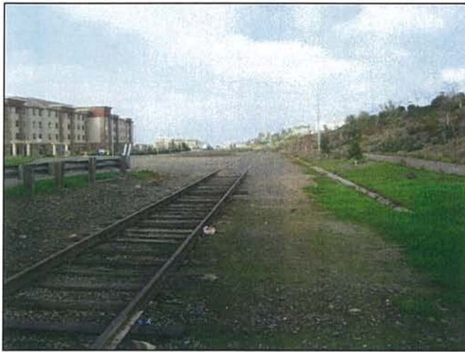
Photo at mile post 116 from US HWY 50 undercrossing. Facing N. Frame 3298
