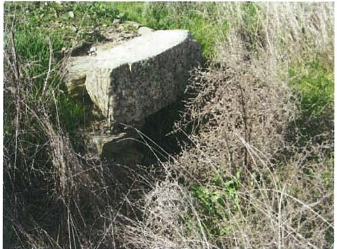
Feature 78: This feature is a stacked greenstone culvert. Facing NW. Frame 3478.
