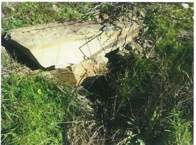
Feature 80: This feature is a stone culvert. Facing E. Frame 3482.
