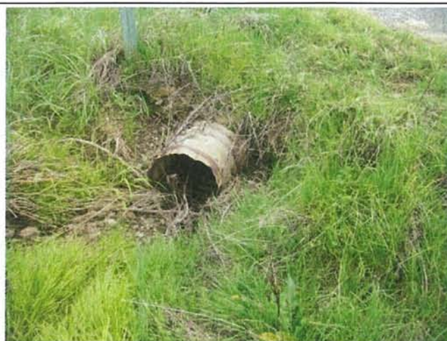
Feature 2: This feature is a corrugated metal culvert. Facing S. Frame 3337.
