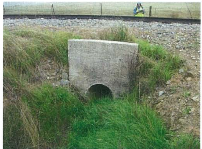
Feature 12: This feature is a poured concrete culvert. Facing NNW. Frame 3316.
