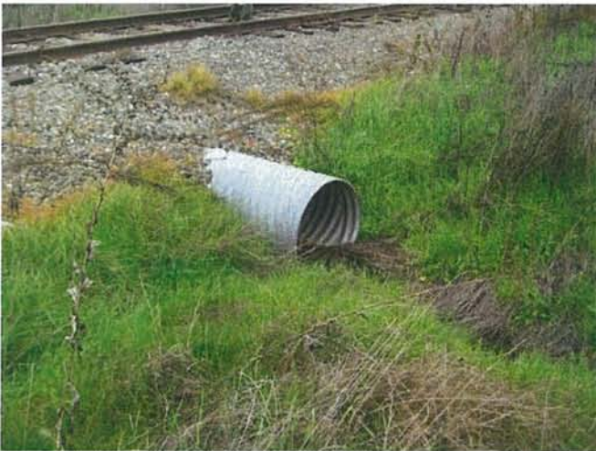
Feature 23: This is a copper steel galvanized culvert. Facing W. Frame 3331.
