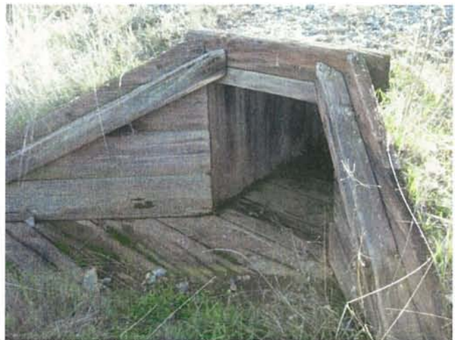
Feature 28: This feature is a large square wooden culvert. Facing S. Frame 3349.
