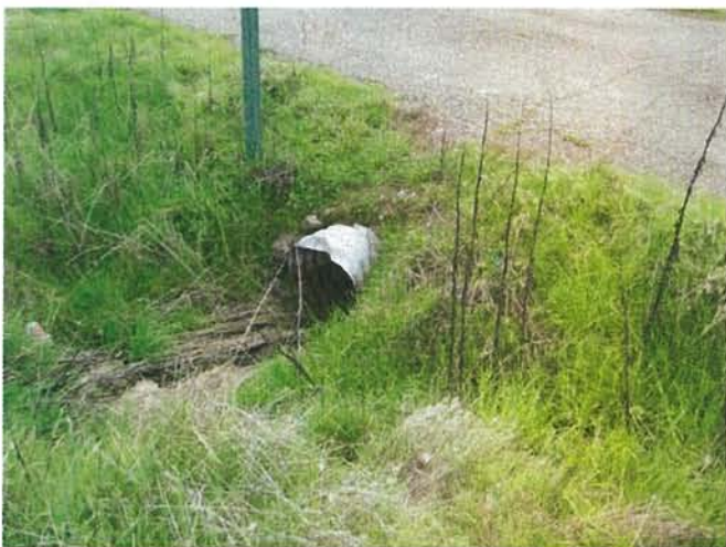
Feature 3: This feature is a corrugated metal culvert. Facing S. Frame 3339.
